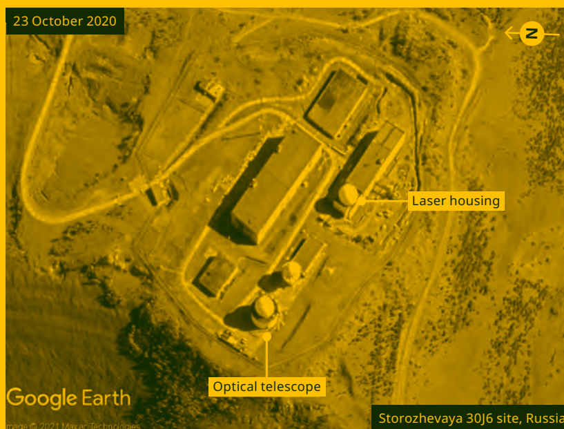
FIGURE 15-47 – KRONA 30J6 OPTICAL COMPLEX NEAR STOROZHEVAYA
